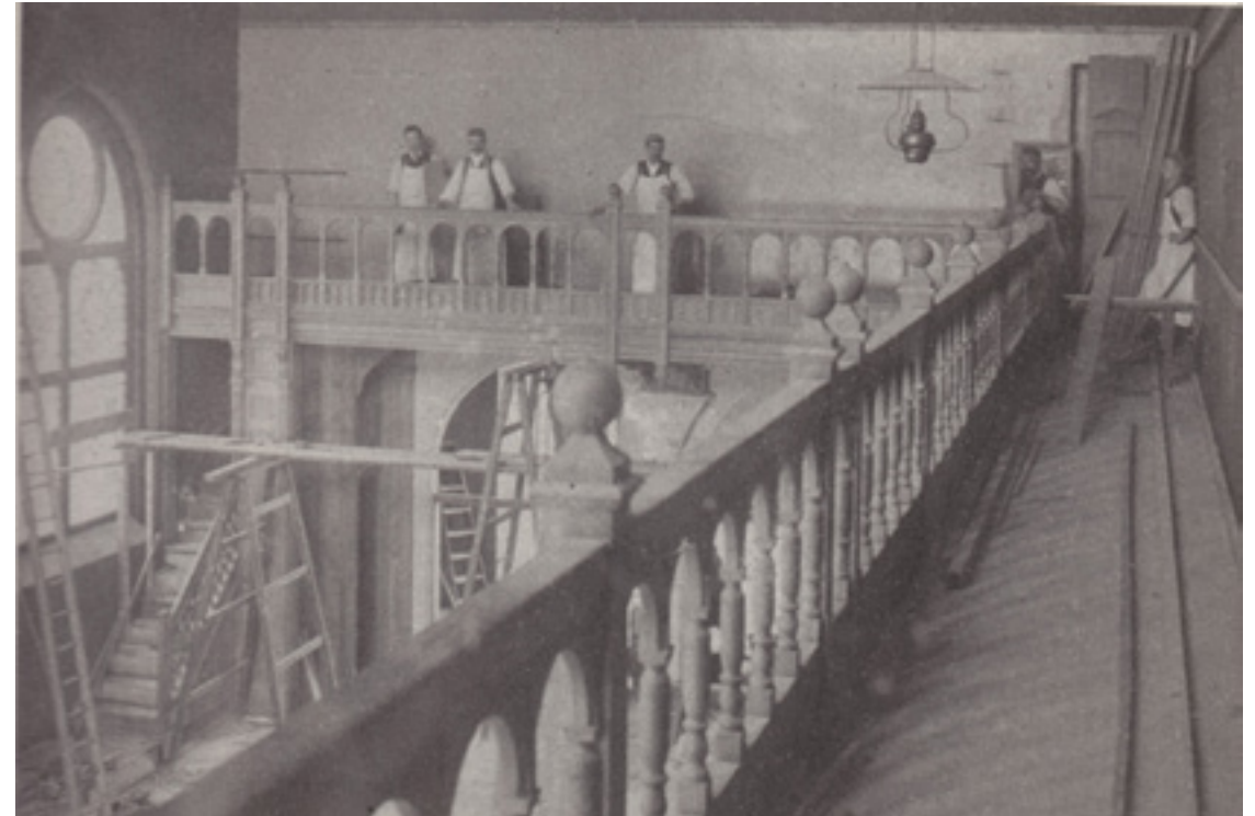
Library under construction
