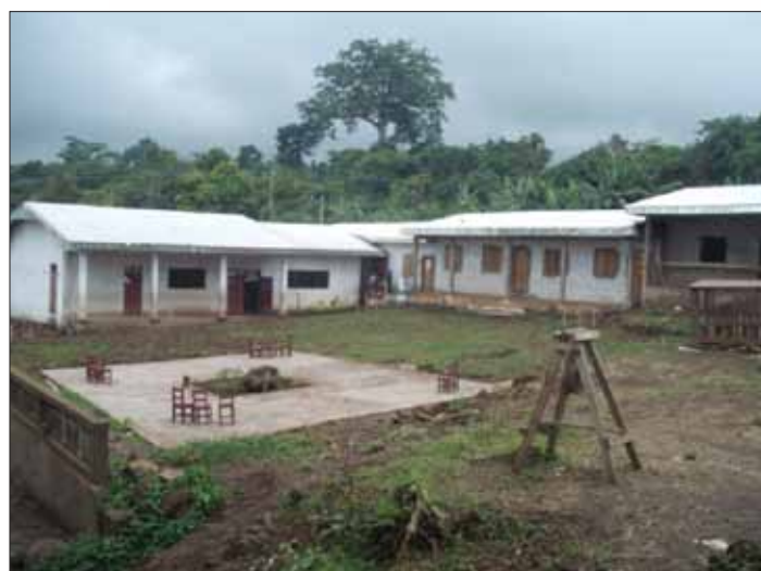
Transforming Jamadianle School: the first stages of the Eden Project
