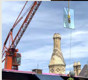
The glass panels for the new Quad roof were lifted into place by crane.
