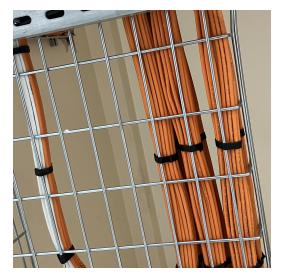
Figure 6: Horizontal Network Cable Basket
