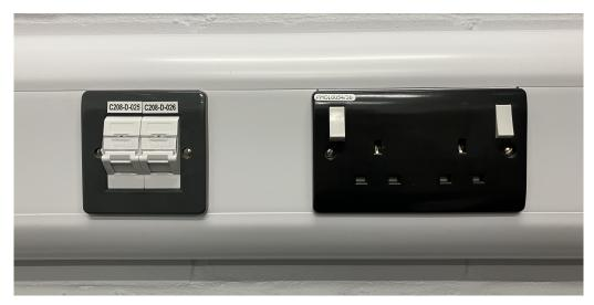
Figure 5: Double Network Socket with Power in Dado Trunking
