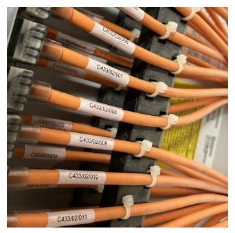
Figure 17: Cables Labelled at Patch Panel
