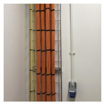
Figure 4: Cable Contained in Cable Basket
