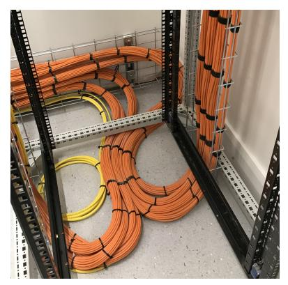
Figure 13: Cable Entry into Bottom of Cabinet
