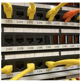
Figure 10: Copper Patch Panel
