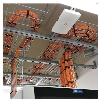
Figure 12: Cable Entry into Top of Cabinet
