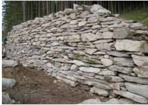
The wall during construction.
