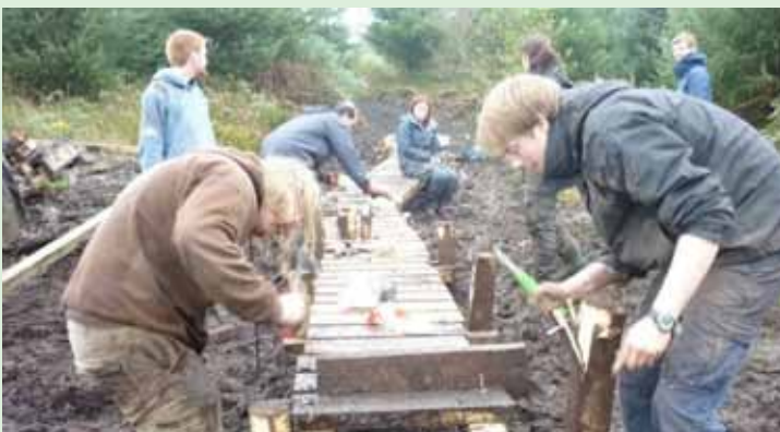
ACV building a boardwalk at Green Phoenix
