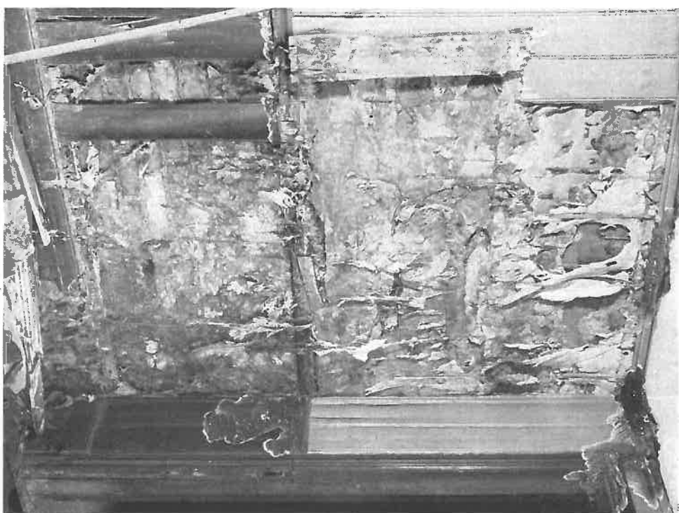
FIG. 1. SEVERE CASE OF DRY ROT IN MATCHBOARDING CAUSED BY Merulius lacrymans
